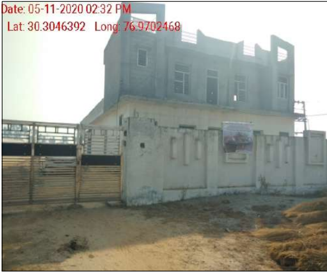
Physical Location: Outside of the Firm (Site 1, On-site Assessment)
